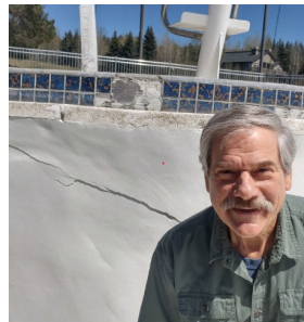
President Dave Galloway Reviews Village Pool Damage
